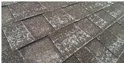
Example of Shingle with high grade granular loss:
